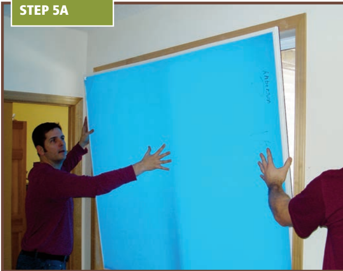
"Dry Fit" of Climate Seal Window Inserts
