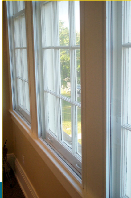
In-jamb mounting style used for both exterior windows and for window above door.
